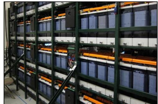
Urban Electric Power's 50kWh nickel-zinc flow battery system being demonstrated at a City University of New York building and supplying electricity to the building during peak electric demand.
